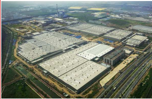
Start of large Shenyang2 plant, China 2012
