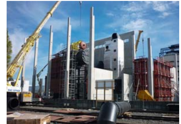
Construction of a wood-fired boiler at the plant in Cholet, France.
